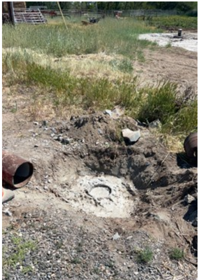
Abandoned and new well in North Central Oregon
