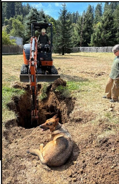
German Shepherd overseeing a landowner permit well installation
