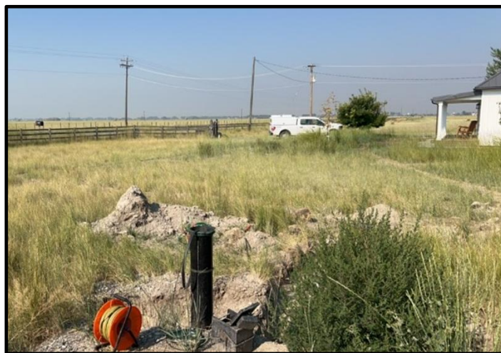
New well near Baker City
