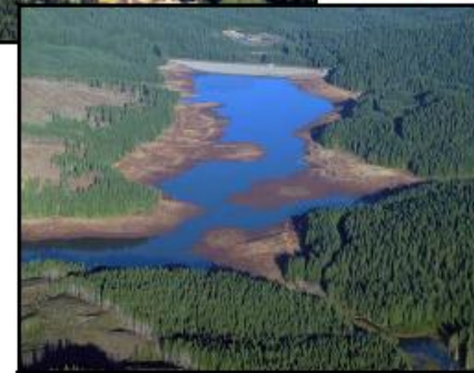
Barney Reservoir, after drawdown, September 2011
