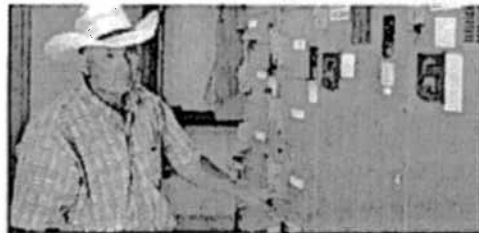
Ed Combs discusses the pumping process for stock water, even though the rest of it has been shut off. H&N photo by Steven Siton
