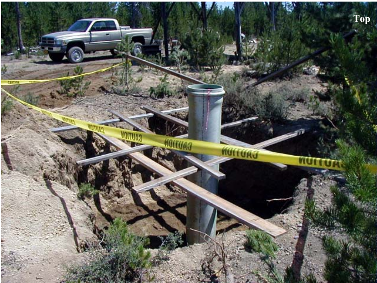
Well dug with backhoe. When well was completed, driller back-filled pit without the benefit of a surface seal. Well casing did not meet standard.
