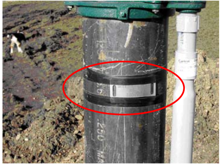
Figure 7. Tag attached with electrical tape.
