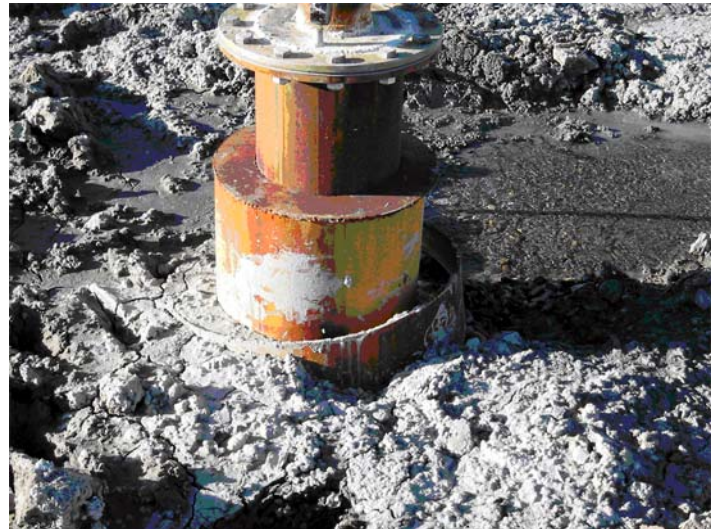
Figure 3. Surface casing left in ground.
