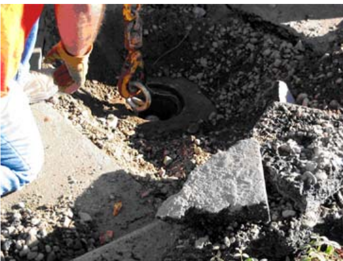
Figure 10. Monitoring well that had been buried in a parking lot.
