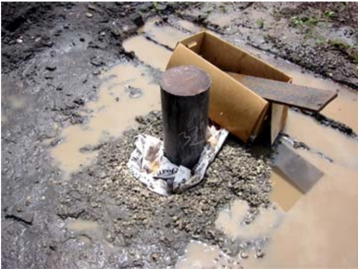
Figure 12. Bentonite bag seal.
