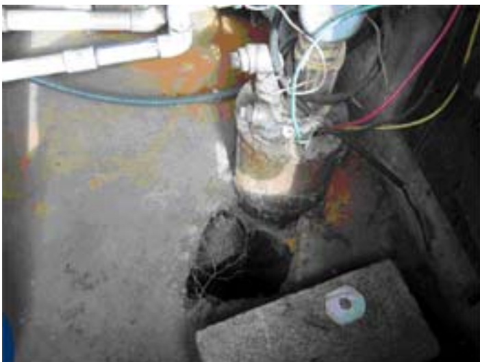
Figure 4. Old well with bad seal.
