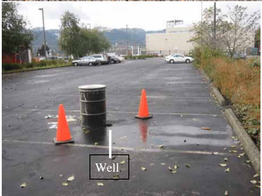
Monitoring Well Left by Driller without a Vault (Barrel was over well).
