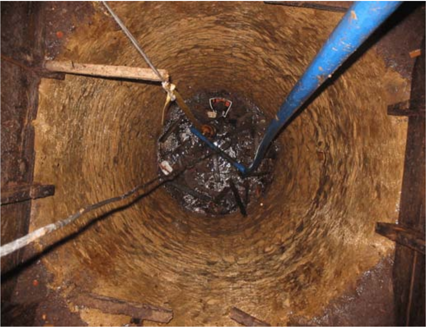
Above - Hand dug well filled with debris. It has since been abandoned.
