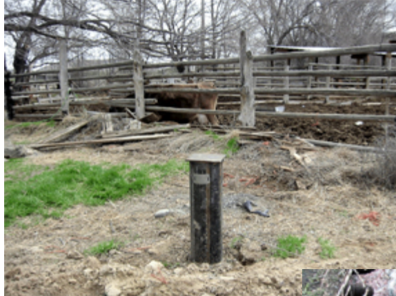
Figure 4. Too close to animal holding area.
