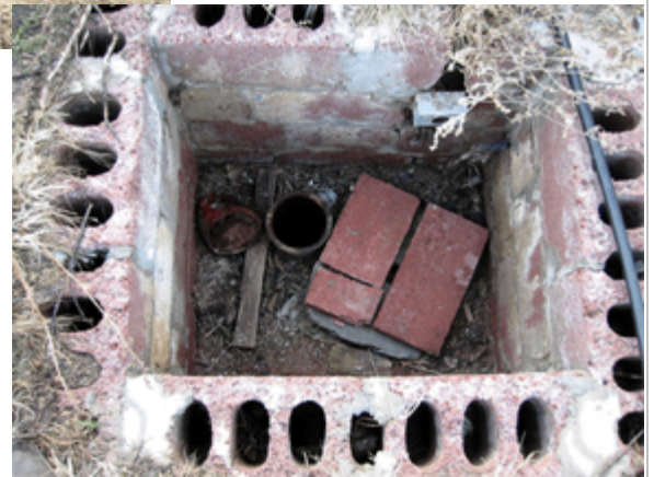
Figure 5. Uncapped cased well in an underground vault.
