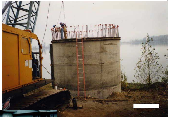
Figure 1: Collector well being installed near the Columbia River.
