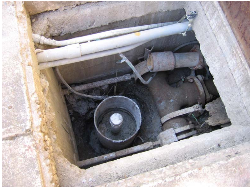
Old water well in a vault being converted into a piezometer.
