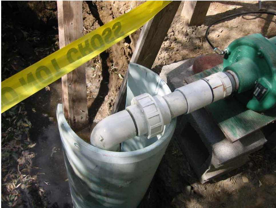
A four year old boy was seriously injured in Eastern Oregon when he fell into this 12"-inch cased water well. The Department worked with the landowner to get the well permanently abandoned.
