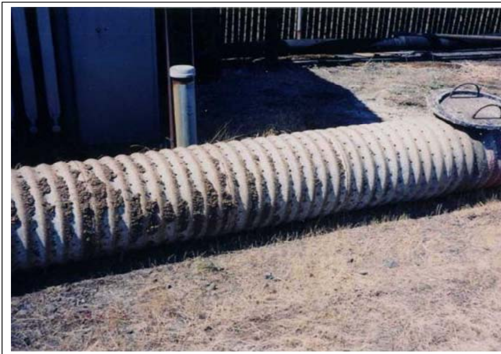
This corrugated pipe remediation well was at a contaminated site in the Portland area. The pipe was removed during the abandonment procedure.
