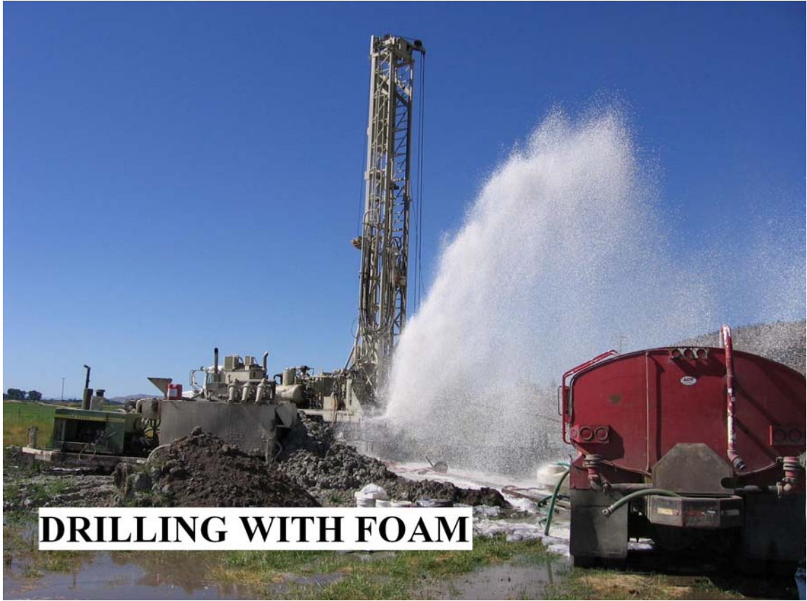
Diesel Truck Being Used As A Pump Motor
