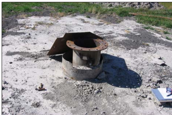
Flange for a Turbine Pump
