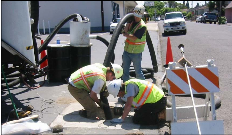
Abandoning a Monitoring Well with a Vac Truck
