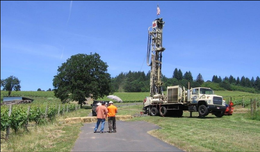
Department Staff inspecting a Water Supply Well being drilled.
