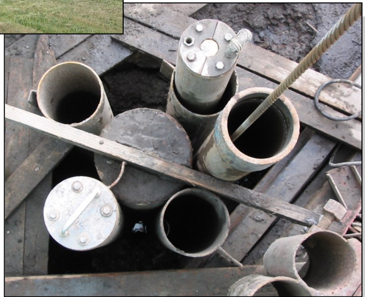
Side-drilling a Water Supply Well in order to replace the Annular Seal.
