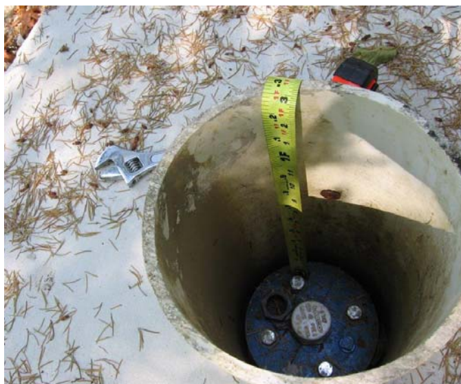
The owner of this well built a well pad over the top. Not only was it very difficult to access, but it also does not meet standards for top terminal height.
