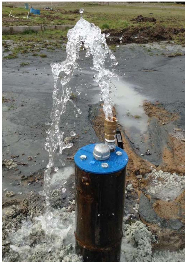
Flowing artesian well with no pressure gauge.
