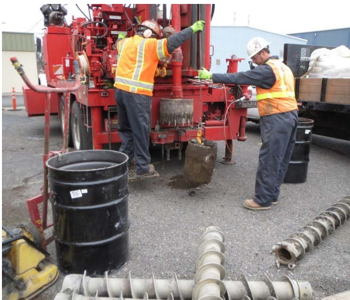
Another monitoring well is abandoned.
