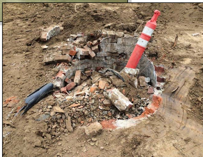
This brick lined dug well was improperly filled with debris during initial grading activities at a construction site. Dug wells must be abandoned by a licensed and bonded driller, or a landowner, utilizing methods approved by the Department.
