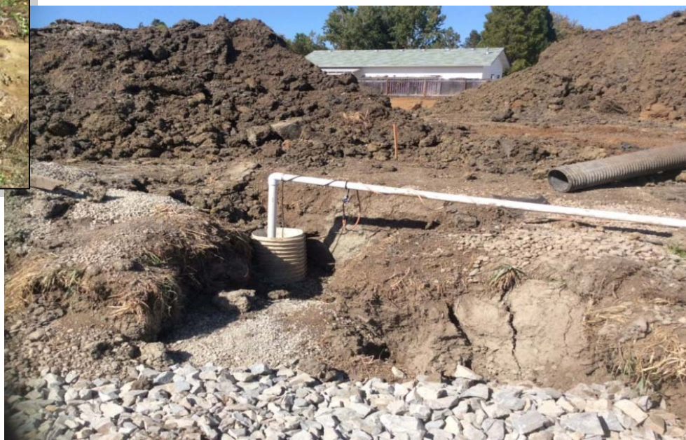
This dewatering well was discovered on a construction site by a regional well inspector. Dewatering wells are water supply wells and must be installed and abandoned by a licensed and bonded driller.
