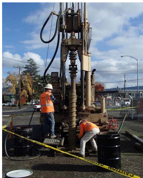
Example — Hollow Stem Auger Drilling Machine.
