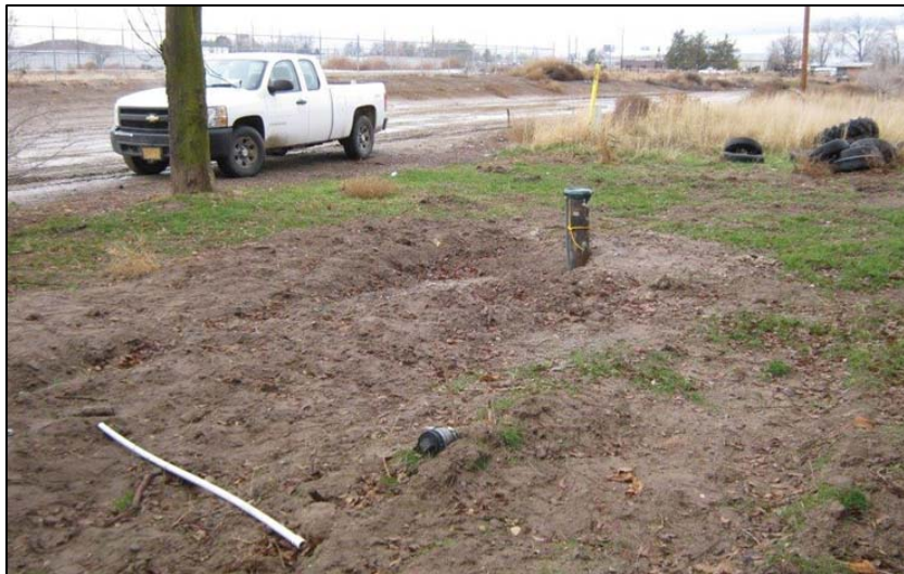
Water Well Installed within 10 feet of a black plastic sewer drain line.
