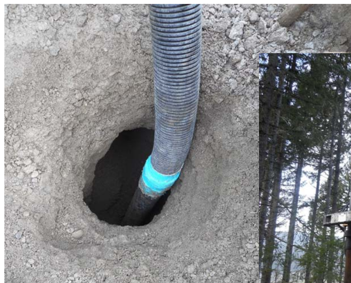
Abandoning a Monitoring Well with a vacuum truck.
