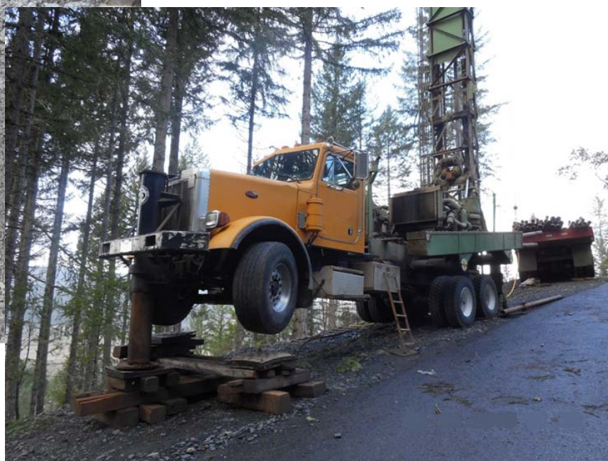
Drilling a Water Supply Well on a slope.
