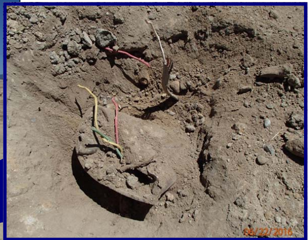
The top of the same Water Supply Well, uncovered following a magnetic search
