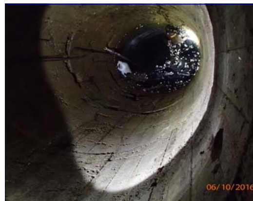
View of the interior of the hand-dug well.
