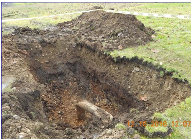
Damaged and buried water well in Southern Oregon.
