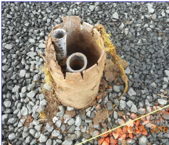
Damaged well at a construction site in Northwest Oregon.
