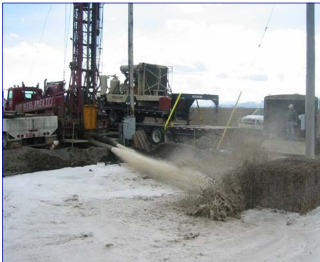
Construction of a well in progress.
