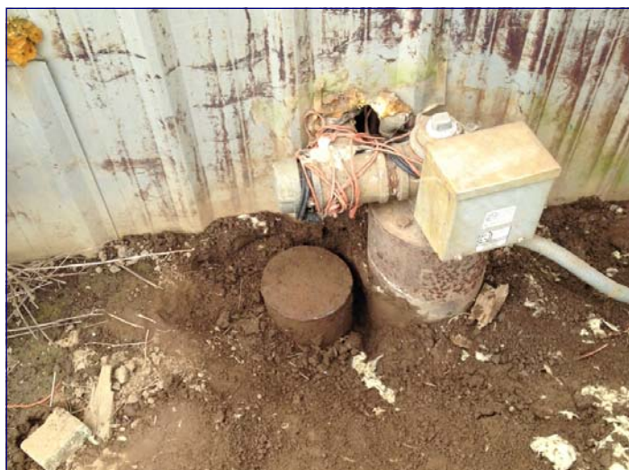
Water well with a large gravel fill tube next to it.
