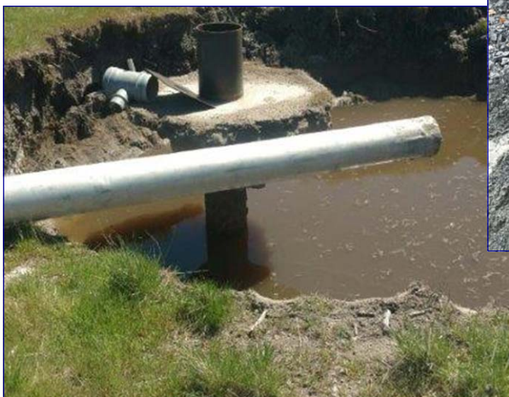
Drill cuttings on the ground flowing towards a creek (in the background).
