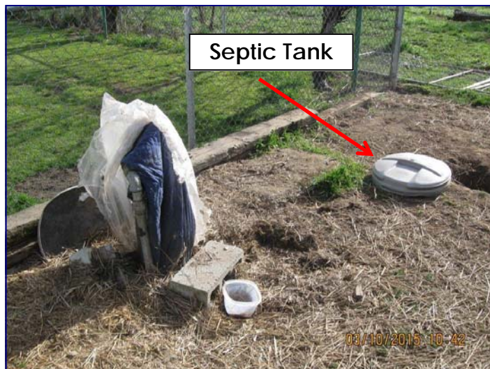
A well too close to a septic tank.
