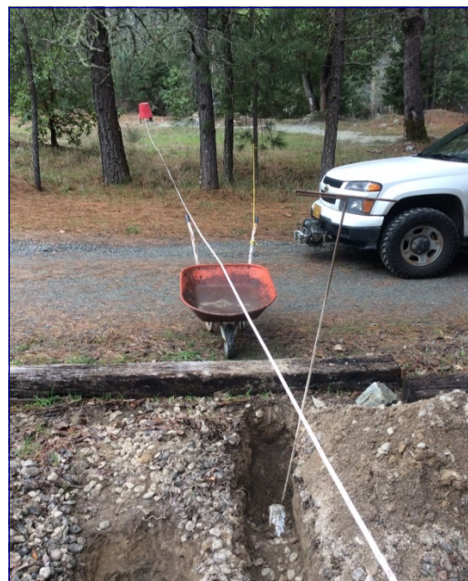
Measuring the leach line distance from a well.
