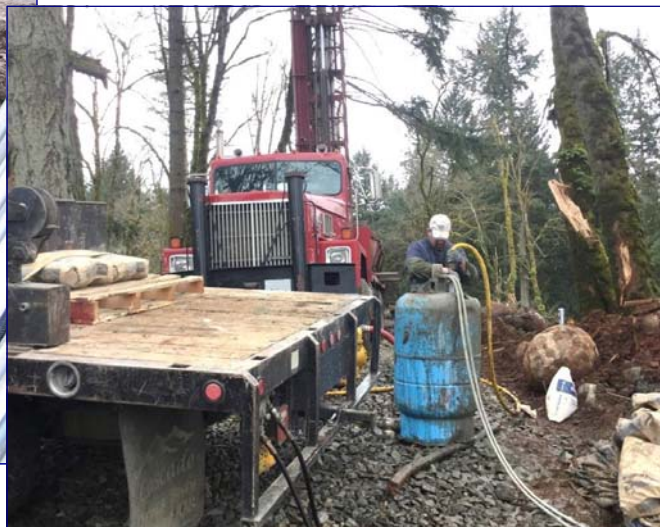
Well constructor mixing cement grout for a well seal.
