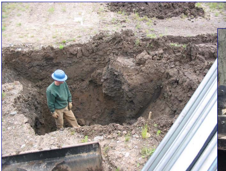
Digging up a buried well on a construction site.
