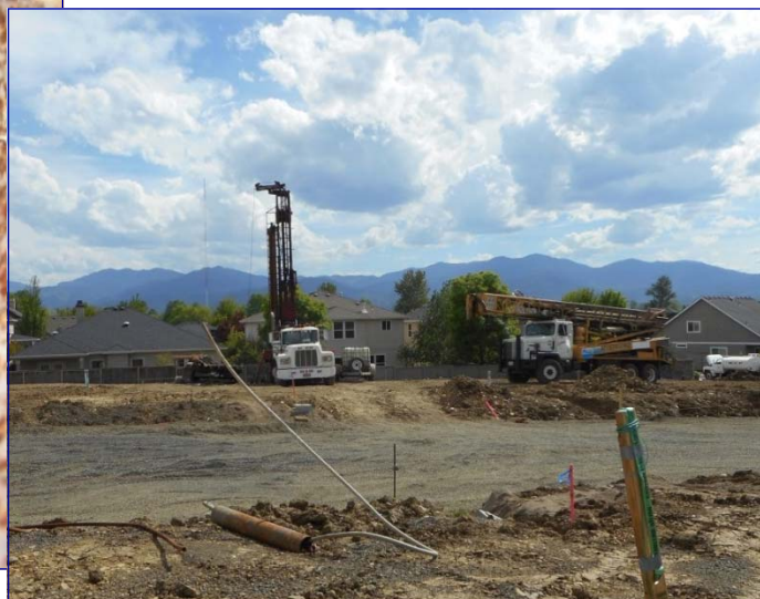
Decommissioning a well on a construction site.
