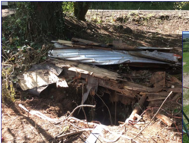
Dangerous hand dug well observed by a well inspector.
