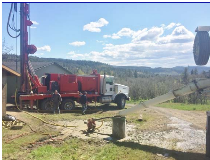
Placing an annular seal in a Mosier area well.
