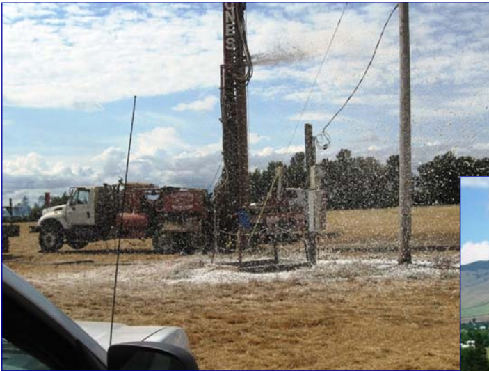
Drilling with foam.
