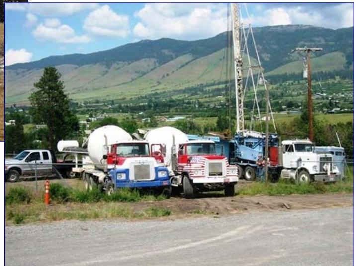
Cement trucks lined up for seal placement.
