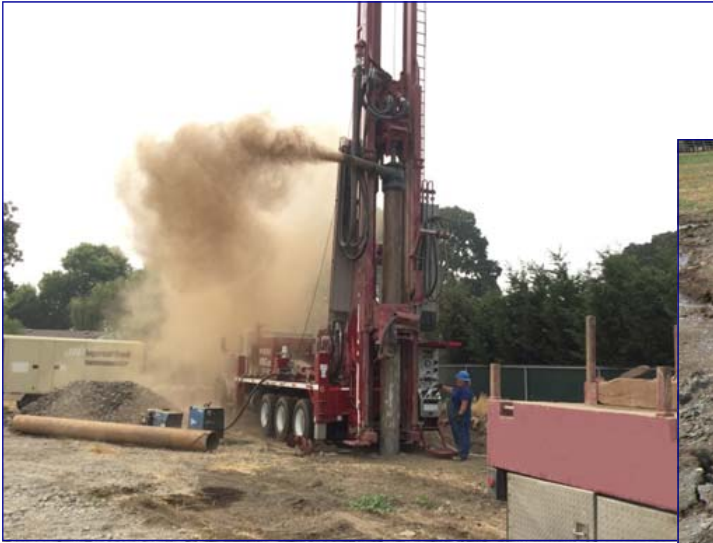
Drilling in progress.
