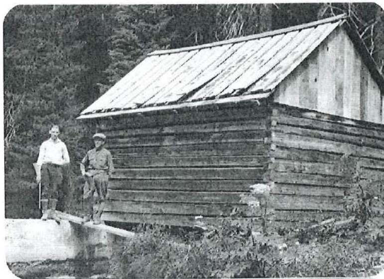
Vic Anderson and Paul Weigelt at Dog River Pipeline Head Gate (8/19/1923)
