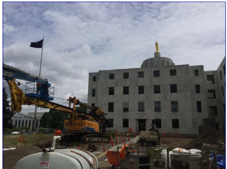
Preparing to drill dewatering wells.
