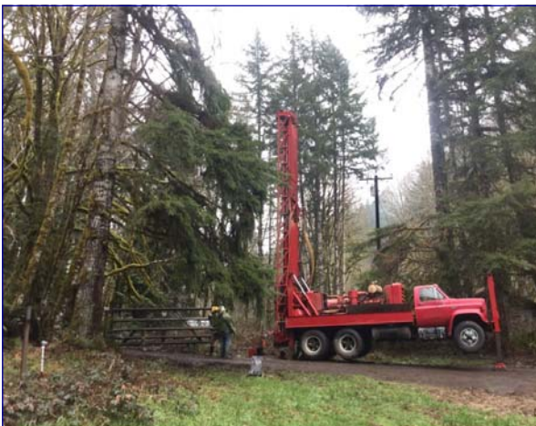
Setting up to repair a well.
