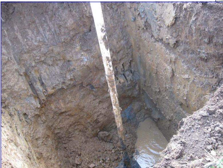
PVC cased well during repair activity.
