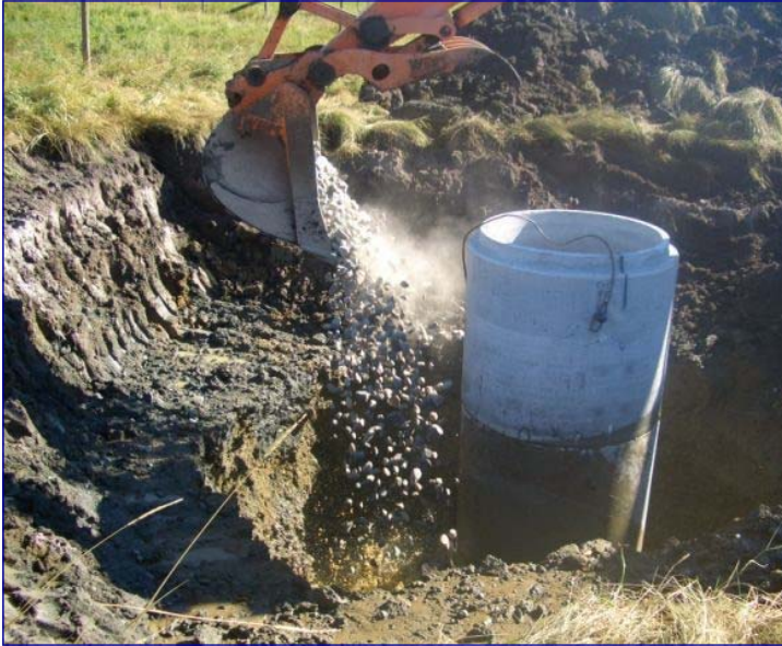
Constructing a dug well.
