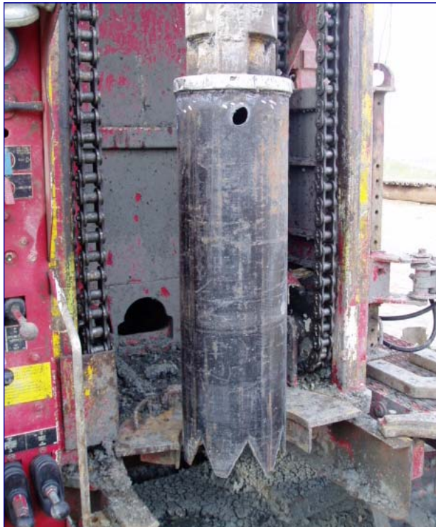
Homemade tool to retrieve broken bit from 1,340 feet below ground surface.
