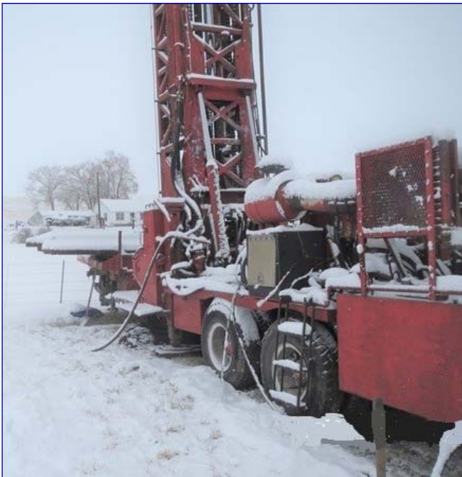
Drill rig set up in the snow.
