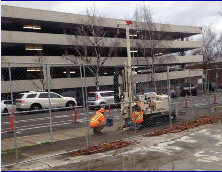
Drilling a geotechnical hole in Salem using a small track rig.
