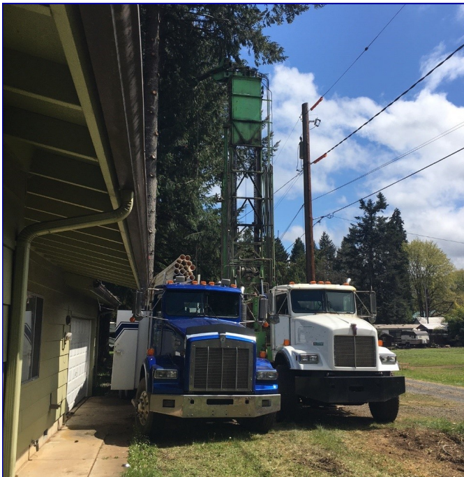
Drilling a well in a tight location.
