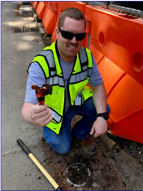
NW Region Well Inspector Tommy Laird inspecting a damaged monitoring well.
