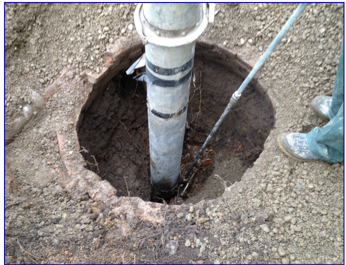
Cleaning out a dug well with a vacuum truck.
