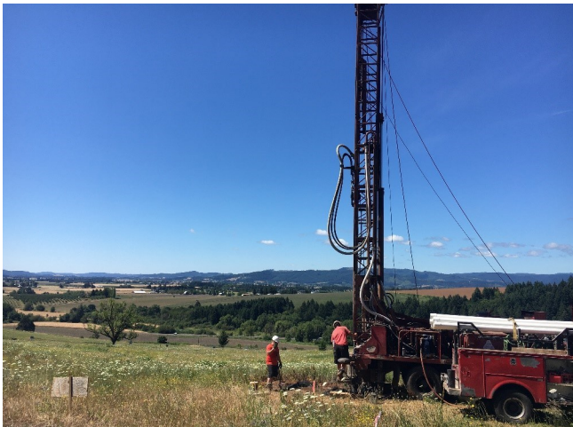
Drilling a well in NW Oregon
