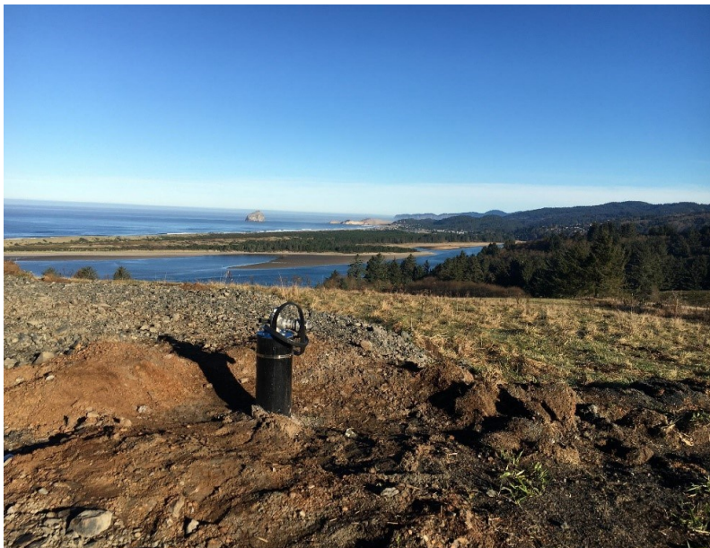
A new water supply well at the coast.
