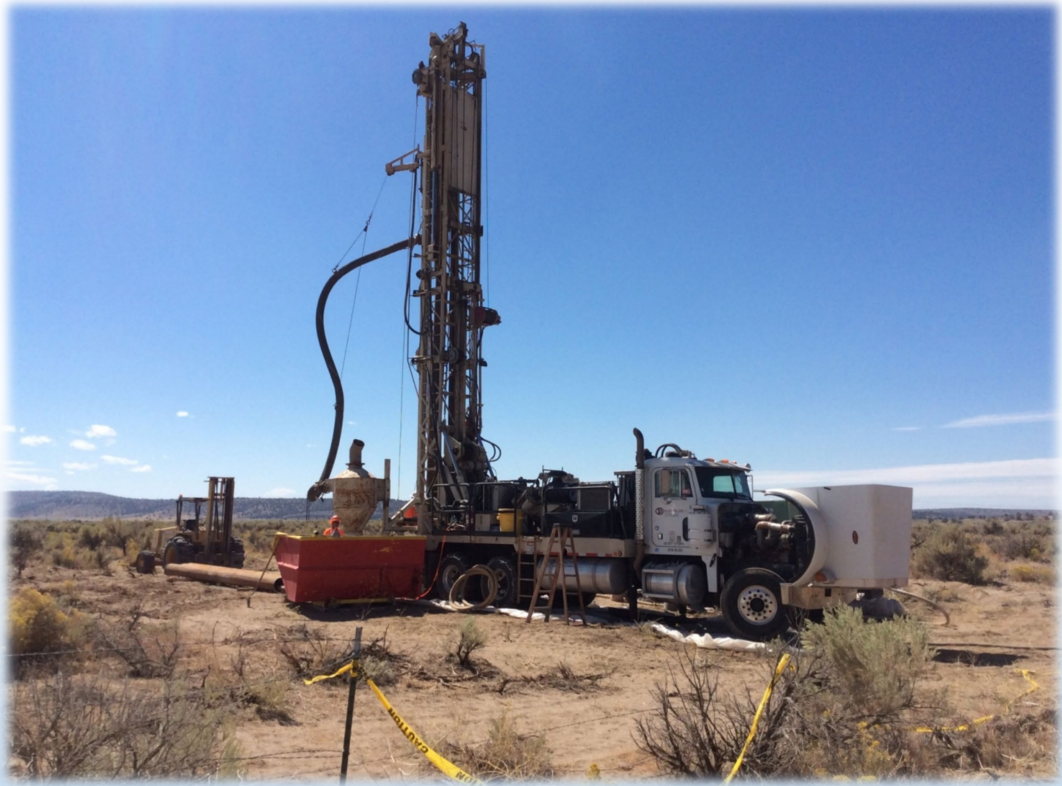
Photo: Drilling a dedicated observation well in the Harney Basin
