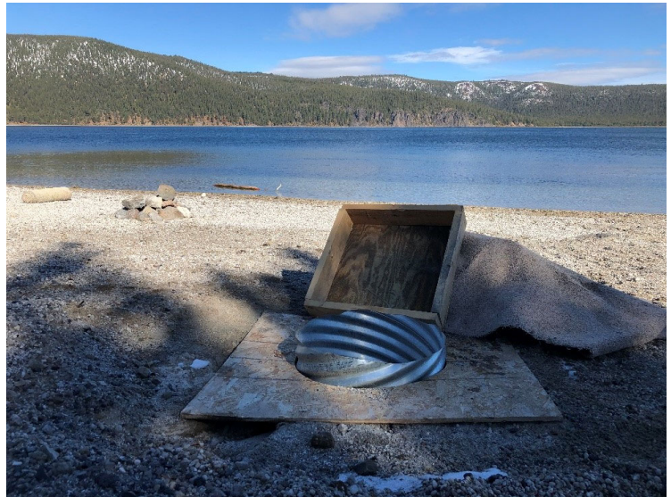
Landowner-constructed well without a permit
