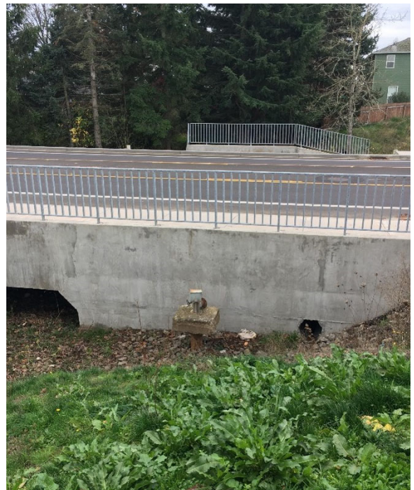
Water supply well to be abandoned
