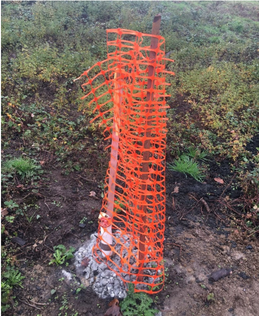
Improperly protected monitoring well
